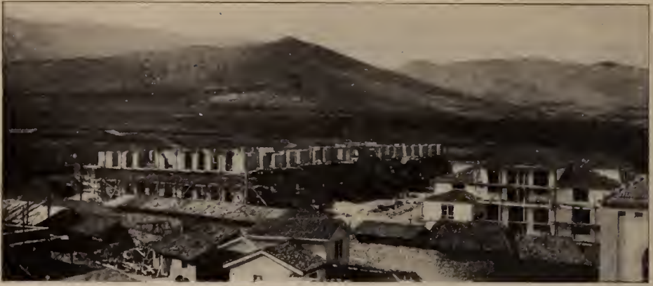
BUILDING THE NEW HOSPITAL AT MARSOVAN
